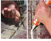
1. Substrate preparation: fastening of loose boards and sealing surface defects
