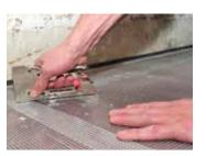
3. Application of KÖSTER Glass Fibre Mesh onto the wooden substrate
