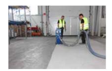
1. The substrate is prepared by shot blasting. Through this process old coatings, as well as contaminated and unstable concrete surfaces are removed down to a coatable layer.
