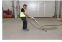
9. After curing, surplus material is removed by vacuum cleaning.
