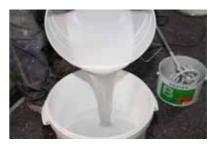
11. To avoid defects due to insufficient mixing, re-pot the material and mix again.
