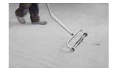
4. When shot blasting is performed with steel abrasive, the surface is cleaned with a magnetic broom. The collected shot can be re-used.
