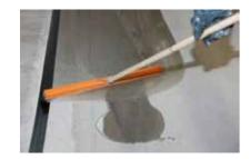
7. KÖSTER LF-BM is used as a primer. Substrates with high vapor drive must be sealed with KÖSTER VAP® 2000.
