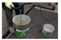
10. The components are mixed for a minimum of 3 minutes with a mechanical stirring device until a homogenous consistency is reached. Follow the mixing procedures given in the Technical Guideline.
