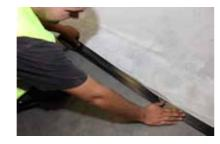
6. Joints and the edges of the work area are taped off to achieve straight edges and to keep the area clean.
