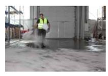
8. Broadcast dried silica sand into the wet primer (only when primed with KÖSTER LF-BM) to increase the bond strength of the subsequent layer.
