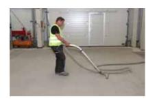
5. To enhance bonding performance all dust and loose particles are removed by vacuum cleaning.
