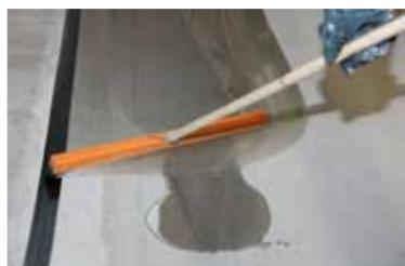
7. KÖSTER LF-BM is used as a primer. Substrates with high vapor drive must be sealed with KÖSTER VAP® 2000.
