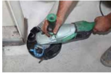
3. Details such as corners and edges have to be prepared by mechanical grinding.
