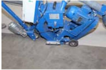
2. Floors and screeds must also be shot blasted to roughen the surface and produce an open pored, absorptive surface.
