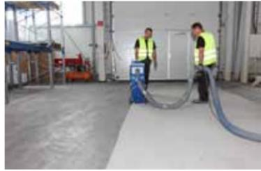
1. The substrate is prepared by shot blasting. Through this process old coatings, as well as contaminated and unstable concrete surfaces are removed down to a coatable layer.
